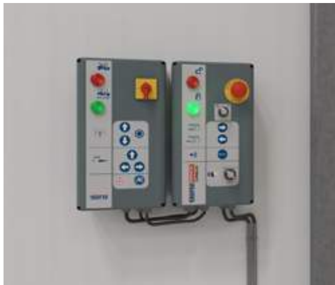
The COMBILOK® G 2 control panel indicator light turns green and signals that the vehicle is safely restrained by the G 2 . The leveller control panel indicator light also turns green indicating that the leveller is in position and loading or unloading can safely commence.
